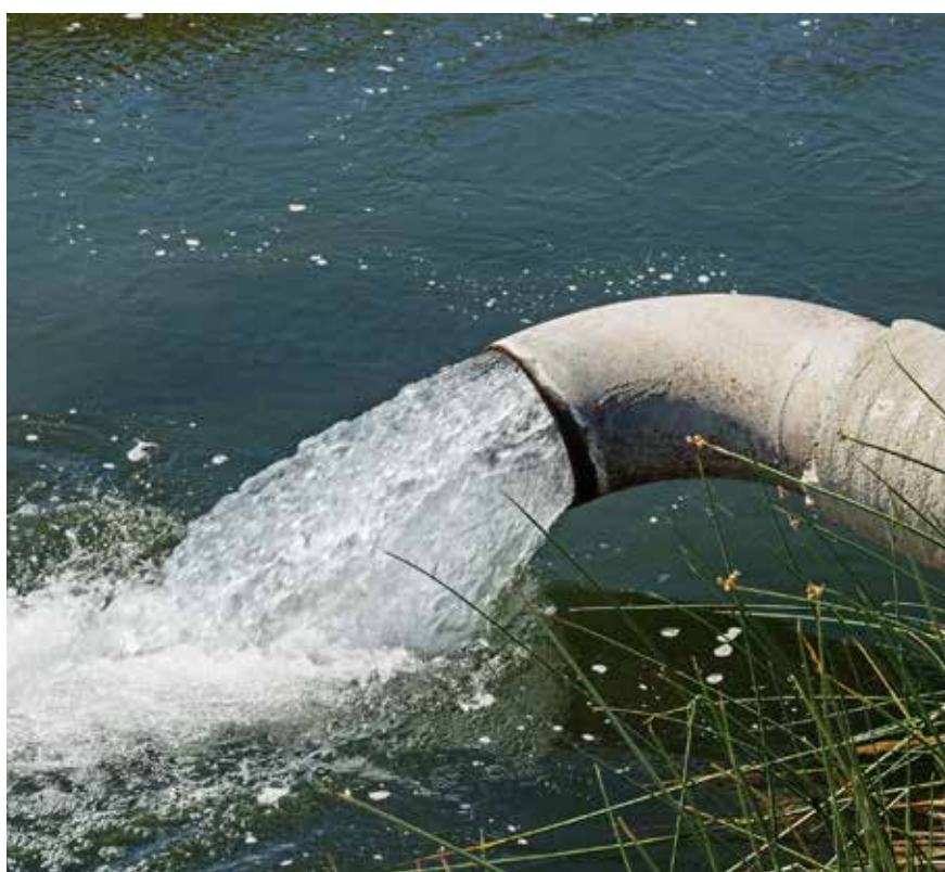
Groundwater pumping out of a pipe into an irrigation canal in California © Community Water Center (CWC)
